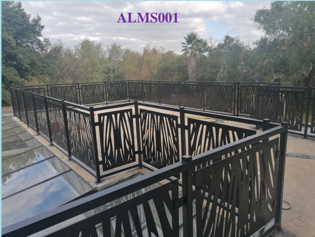
2mm perforated plates fixed to square tubes all round giving a unique look.
