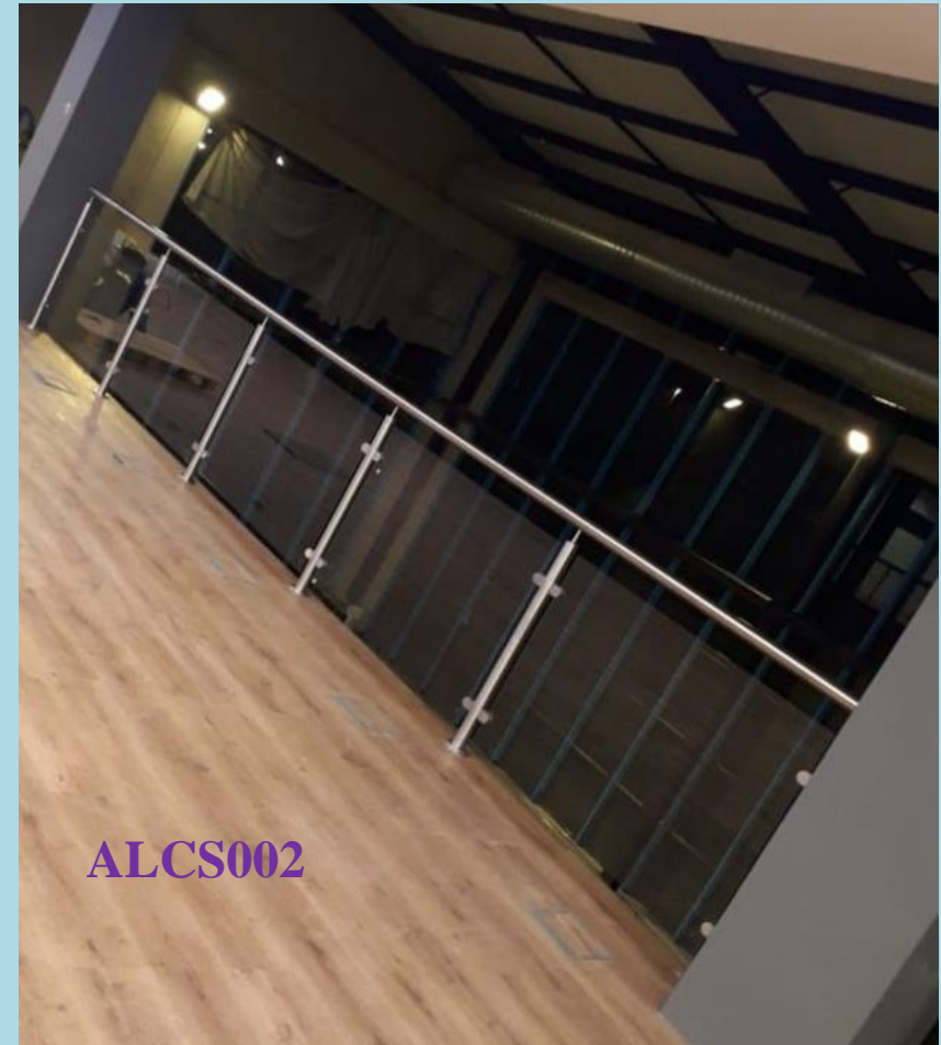
8mm thick toughened glass fixed in a stainless steel frame
