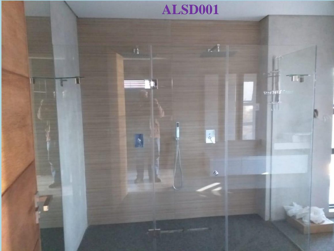
8mm thick toughened glass cubicle
