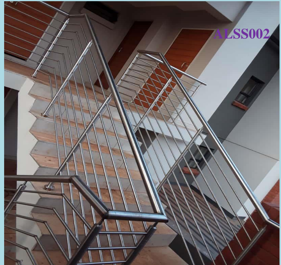
8 Off - Dia 16mm infill rods staircase Also options available in 5 or 6 Off infill rods which are less in price.
