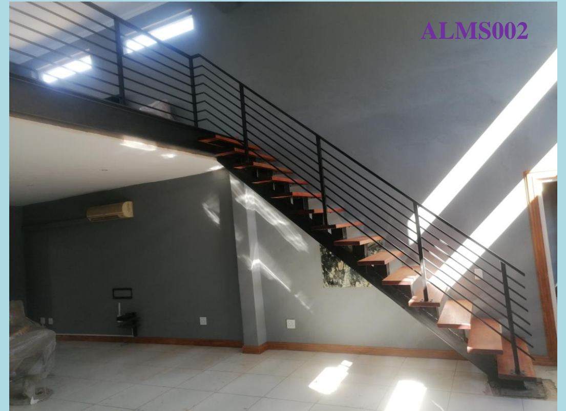
Mild steel beam supported staircase with wooden stair treads and mild steel handrails.
