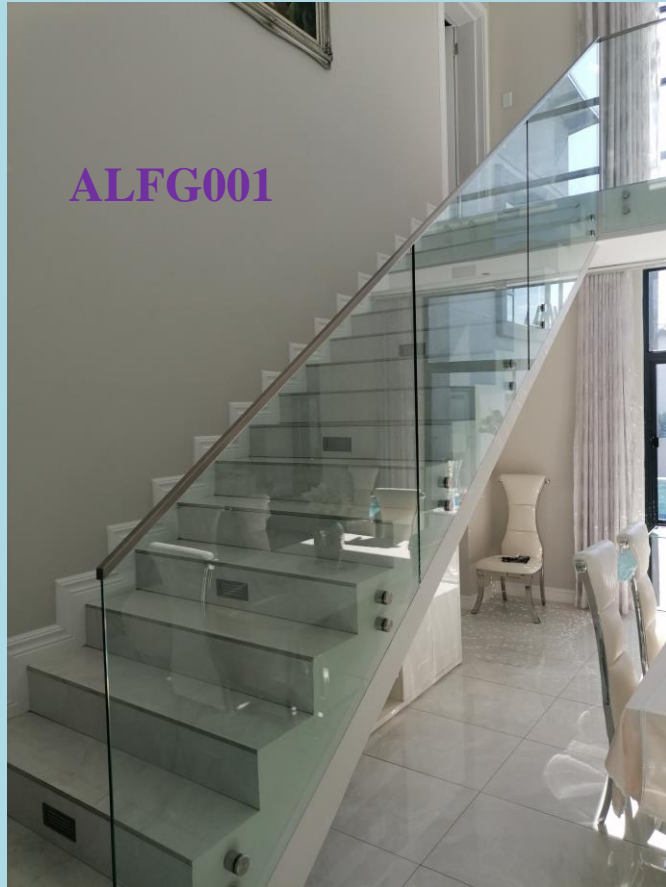
Side Fixed 12mm thick toughened glass Stairs With 20 x 25 slotted silver handrail
