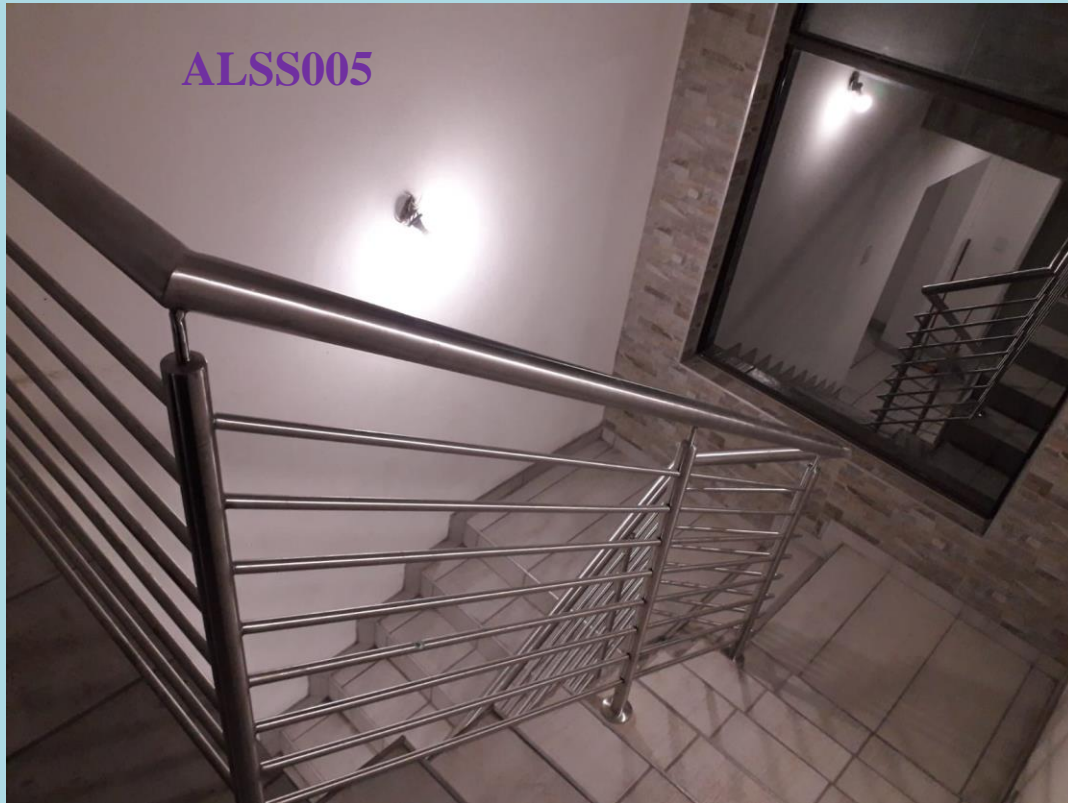
8 Off - Dia 16mm infill rods staircase Also options available in 5 or 6 Off infill rods which are less in price.
