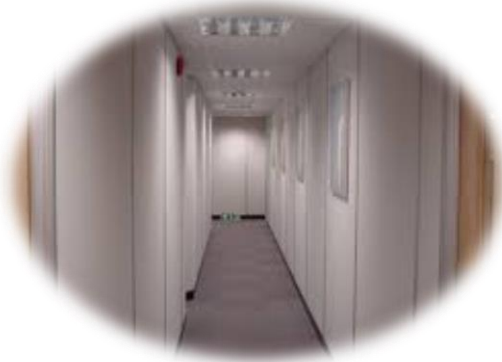
Fire Protected Corridor
